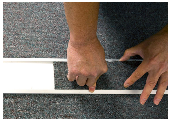
Attach carpet tile to track raceway
